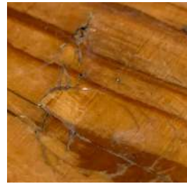
Repair Burns & Dents.
